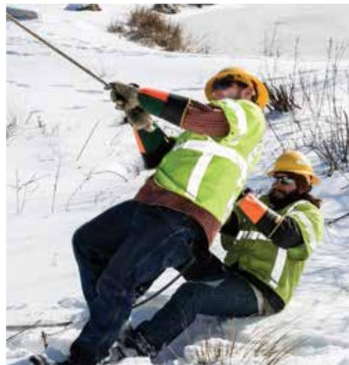
**TEAMWORK:** Linemen Justin Franko, left, and John Farrell join forces on a handline to hoist new conductor to a pole top along Kletsko Road.
